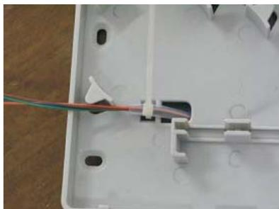
Pic6: dark-routing leads in box and fixes by nylon tie
